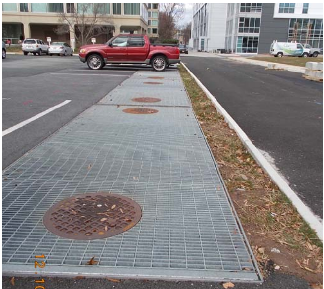
3 EASEMENT WEST OF ALLEY LOOKING NORTH
