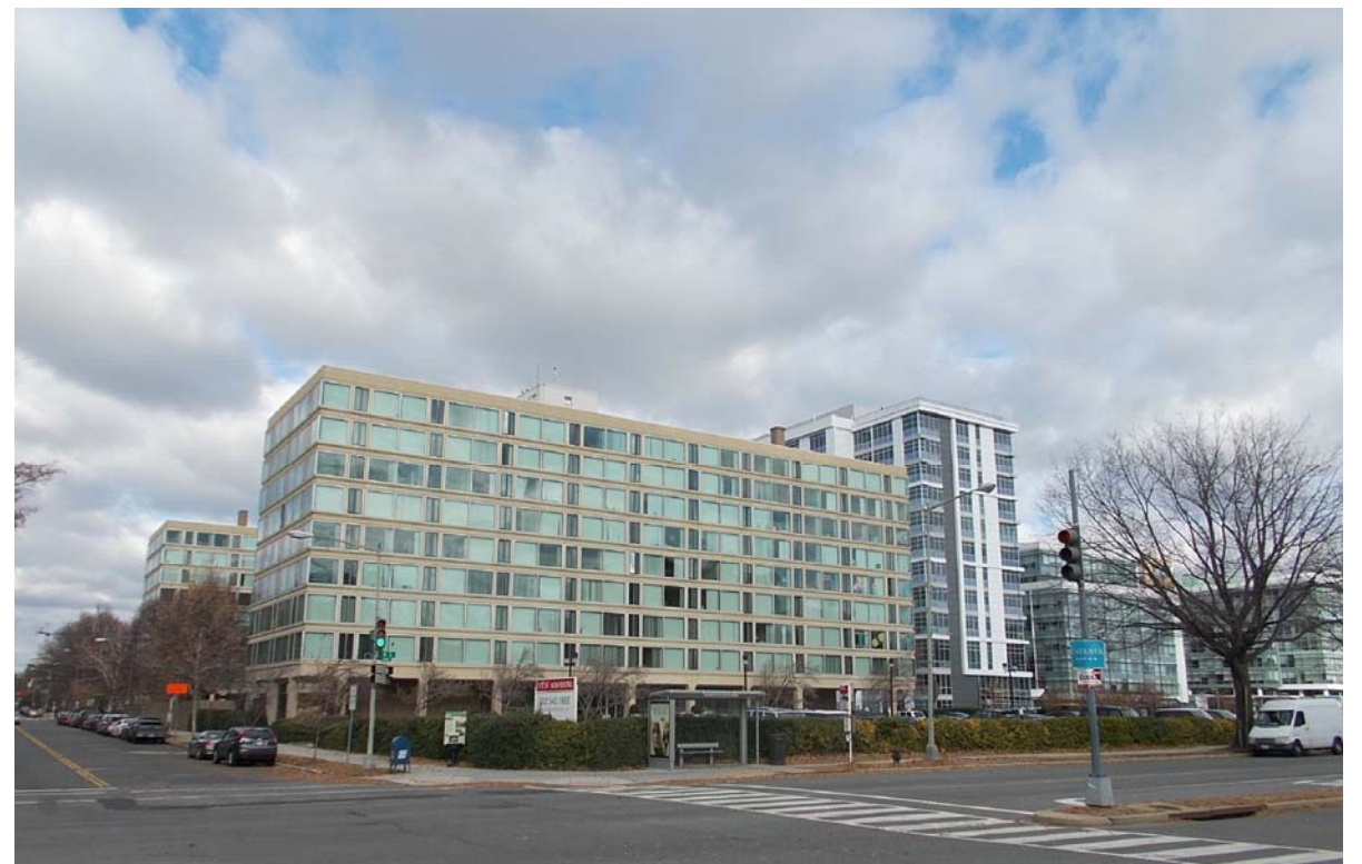
7 VIEW OF M STREET LOOKING EAST
