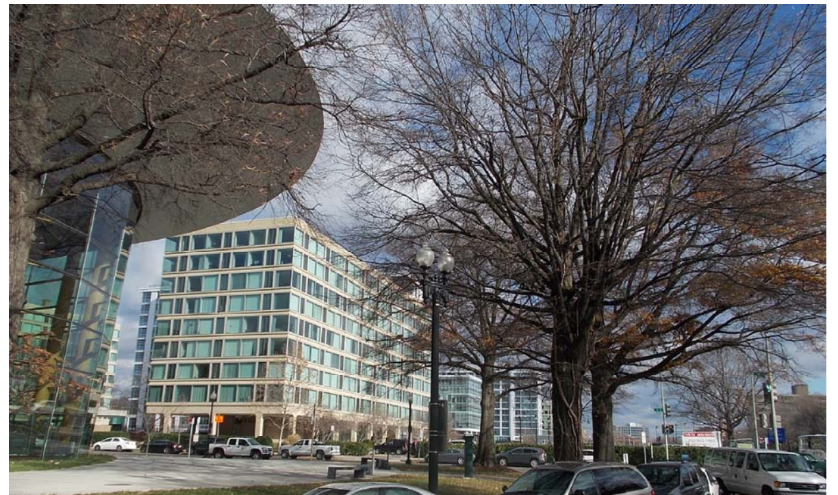
9 VIEW OF SITE WEST ON M STREET WITH ARENA STAGE
