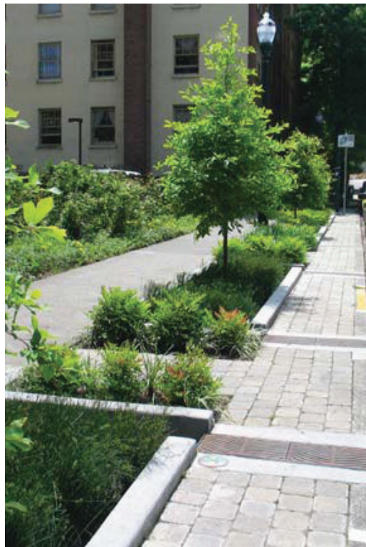
BIORETENTION AT CURB
