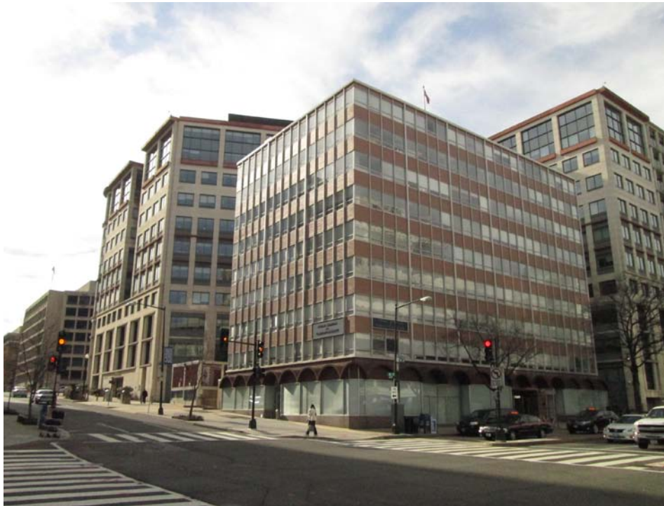
1 K STREET LOOKING SOUTH DOWN 21ST STREET
