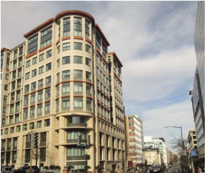
3 PENNSYLVANIA AVE. LOOKING NORTH DOWN 21ST STREET
