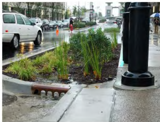
GAP IN CURB DIRECTS STORMWATER TO PLANTS
