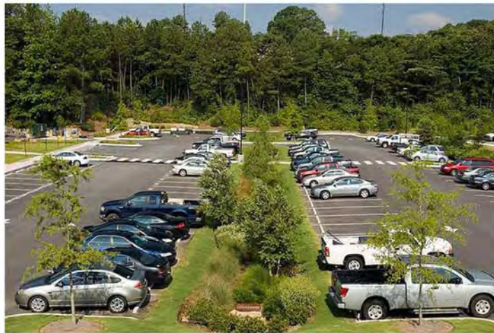
BIORETENTION AREA IN PARKING MEDIAN
