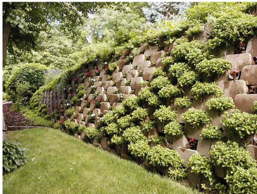
VEGETATED RETAINING WALL SYSTEM
