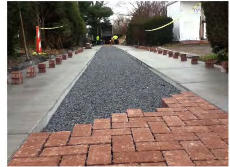
UNIT PAVERS OVER PERMEABLE BASE COURSE
