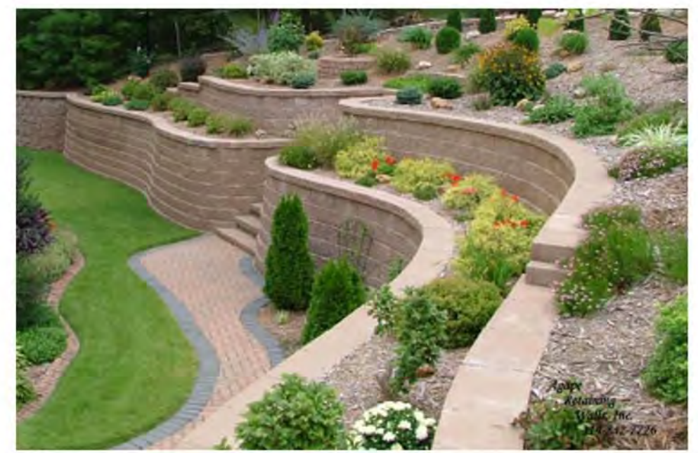
SEGMENTAL RETAINING WALLS WITH PLANTED TERRACES
