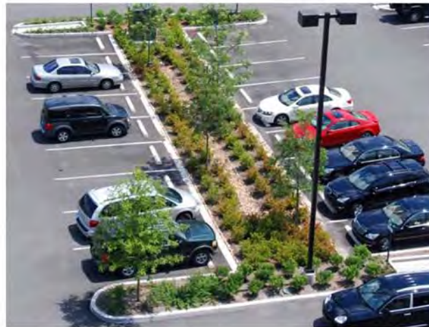
BIORETENTION AREA IN PARKING MEDIAN
