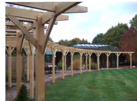
CURVED SHADE STRUCTURE
