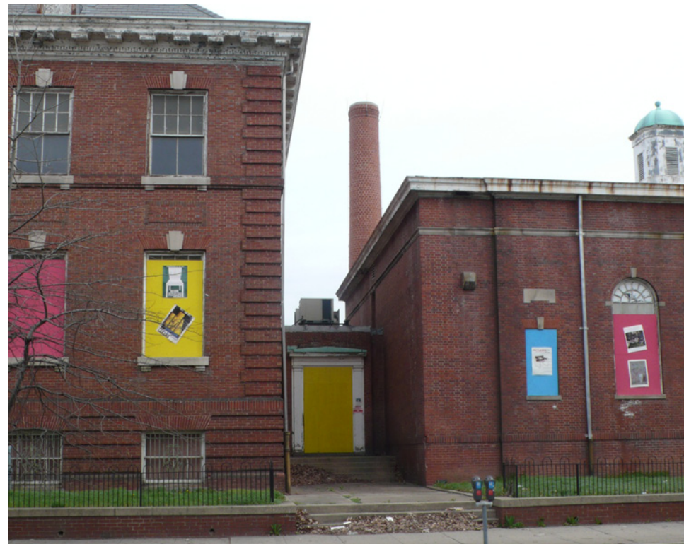
2 - Randall School I Street facade between main building and auditorium
