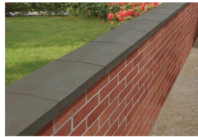
MASONRY PLANTER WALLS
