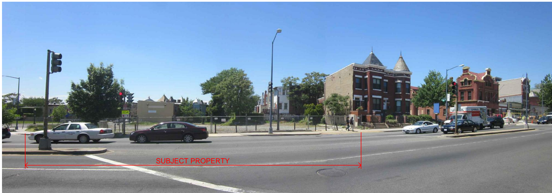
4. VIEW ACROSS NORTH CAPITOL
