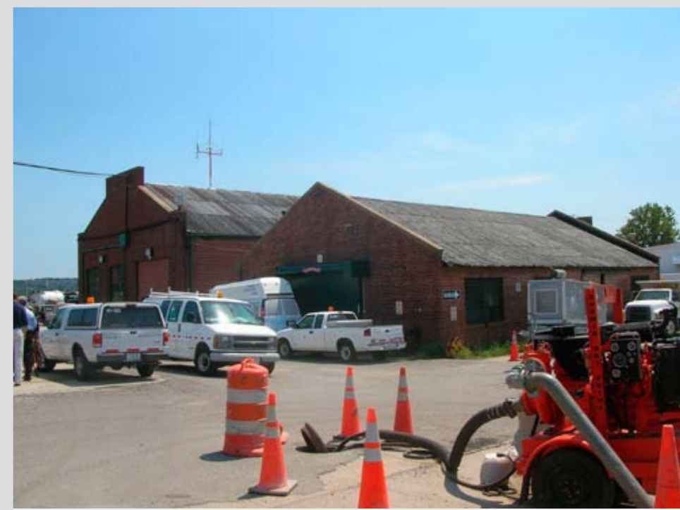
5 CONCRETE PREFAB & CARPENTER SHOP - NORTH ELEVATION
