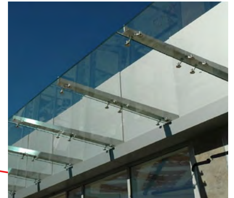
Glass Canopy held with Spider-Fitting Ribs
