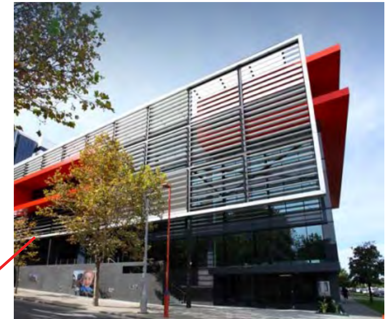
Extruded Metal Cornice
