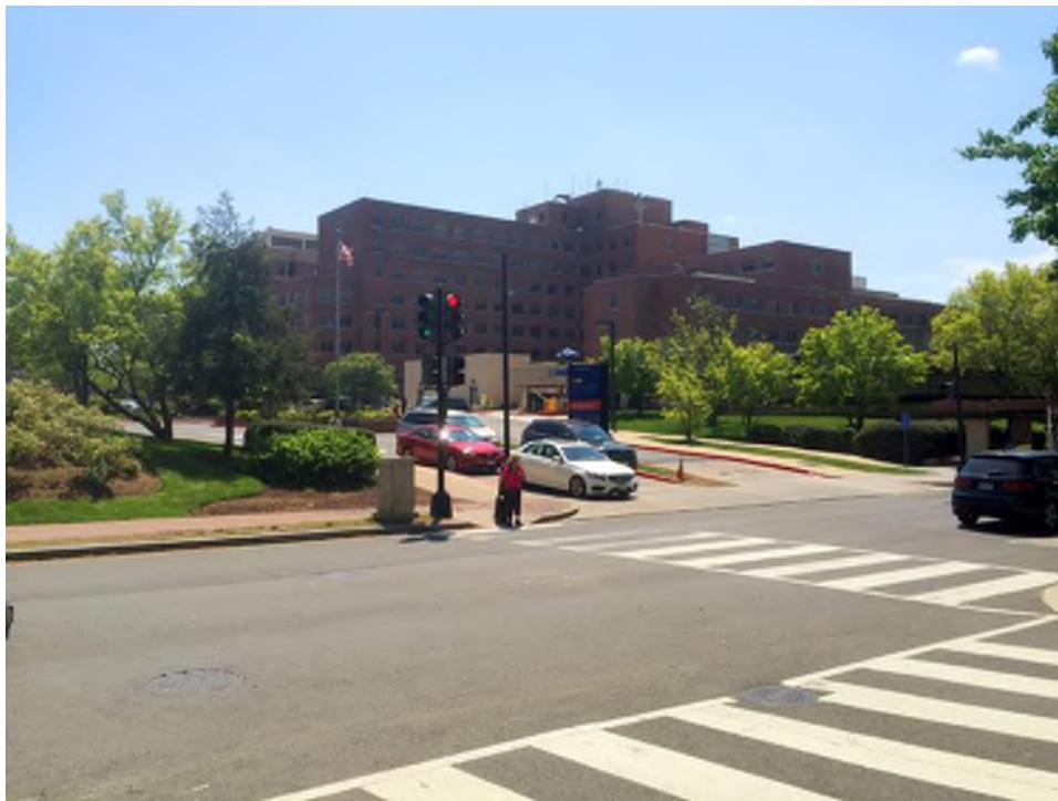
5. VIEW FROM RESERVOIR RD & 38TH ST
