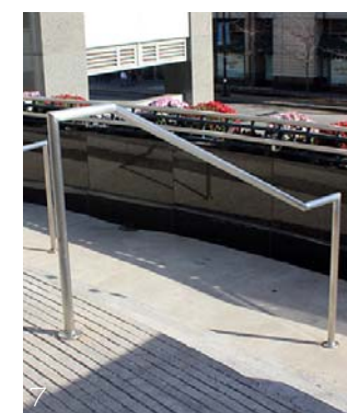
GRAND STAIR RAILING ON MASS. AVENUE
