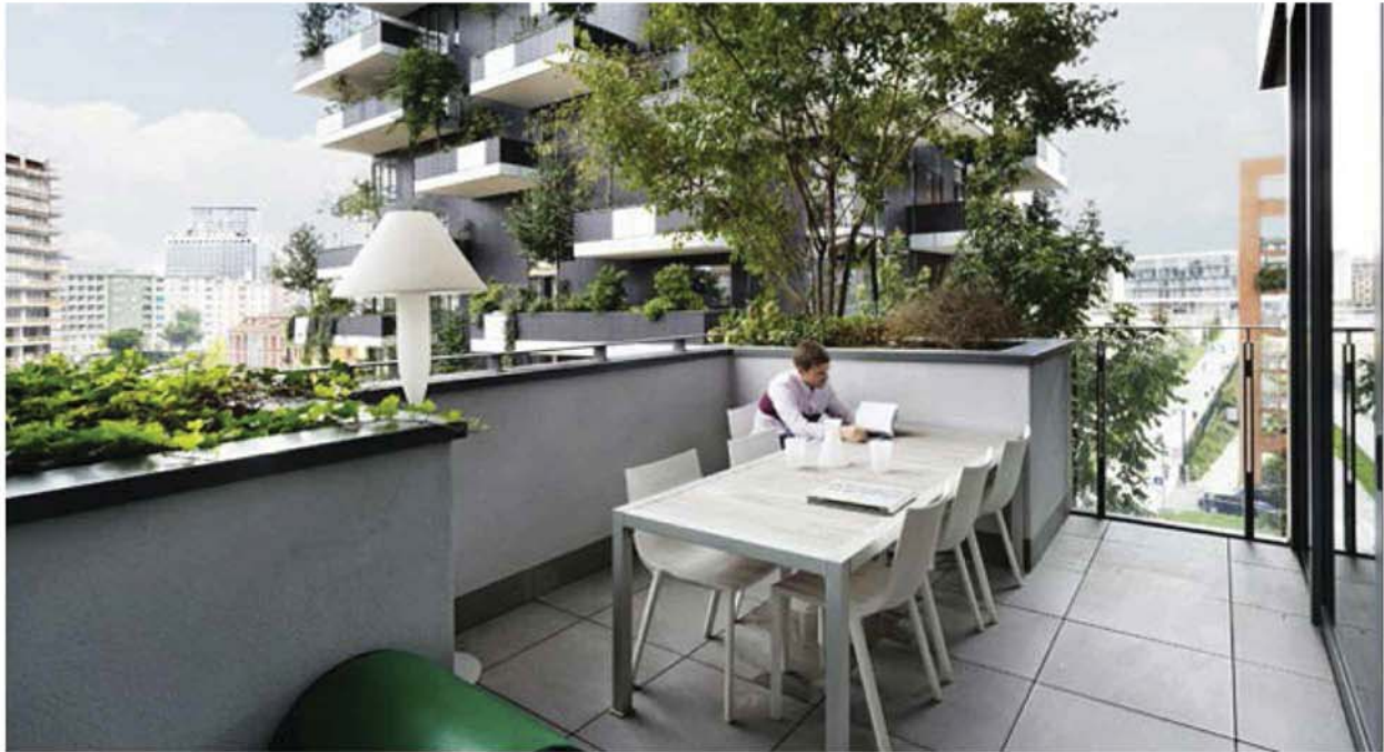
Private Terrace Planter as Divider and Parapet
