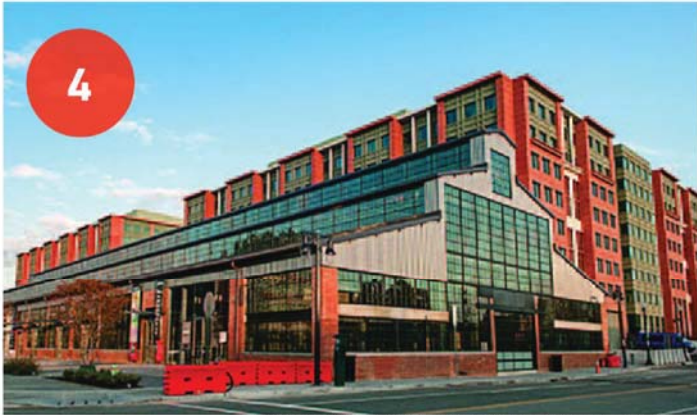
THE BOILERMAKER SHOPS, 300 TINGEY STREET SE - RETAIL BUILDING
