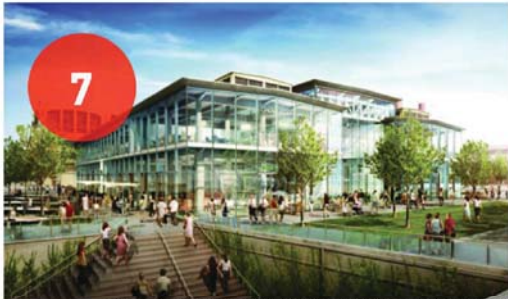
THE LUMBER SHED, 301 WATER STREET SE - RETAIL BUILDING
