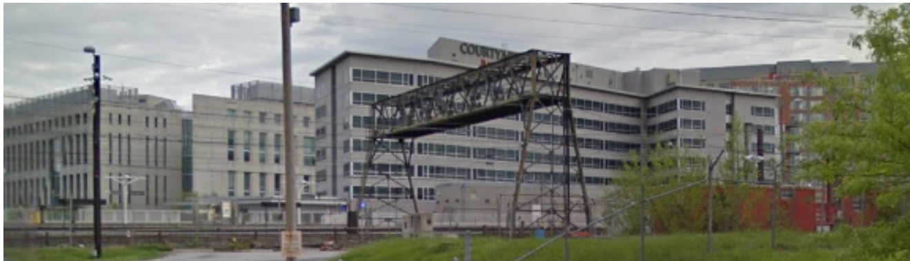
9 - VIEW OF RAILROAD SIGNAL BRIDGE FROM 3RD STREET
