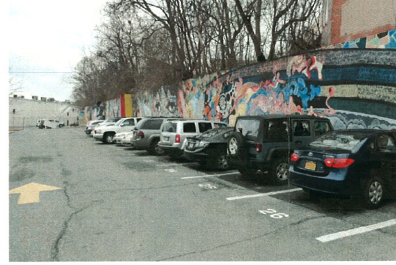
F. Retaining wall
