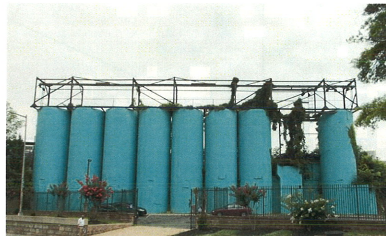
J. Silos on Rhode Island Ave.
