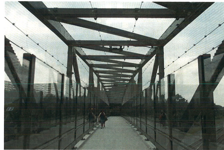
F. Metro Bridge
