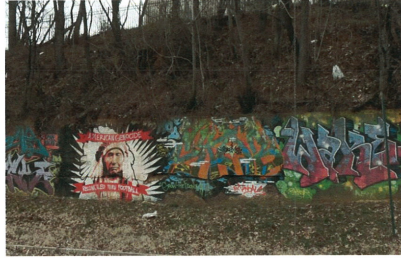
E. Retaining wall
