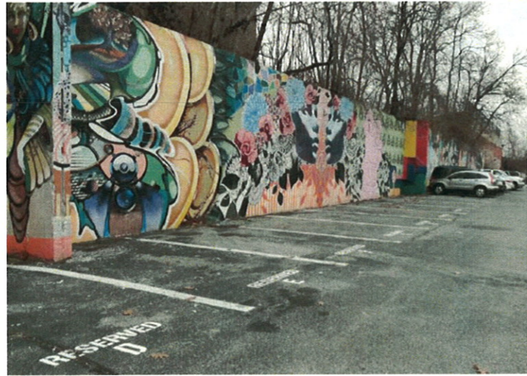
D. Retaining wall
