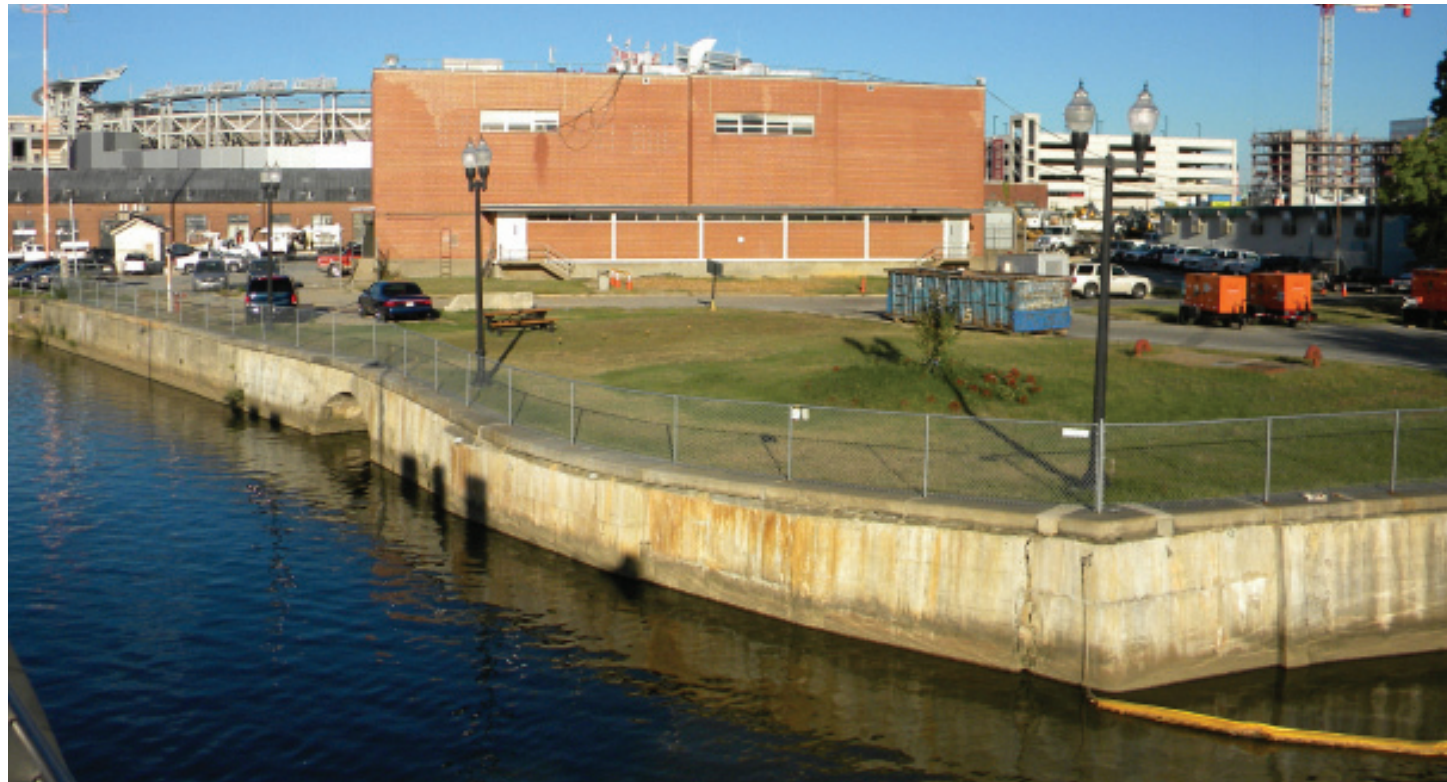
VIEW FROM ANACOSTIA RIVERWALK TRAIL - FACING NORTHWEST
