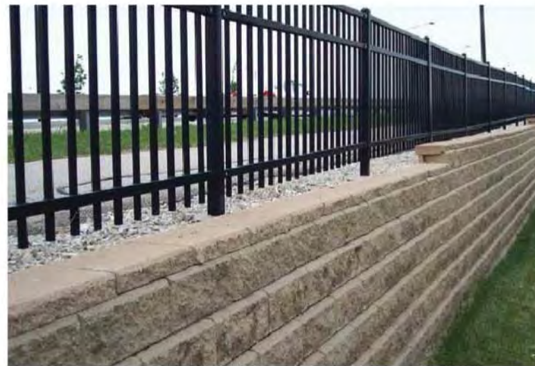
RETAINING WALL WITH GUARDRAIL
