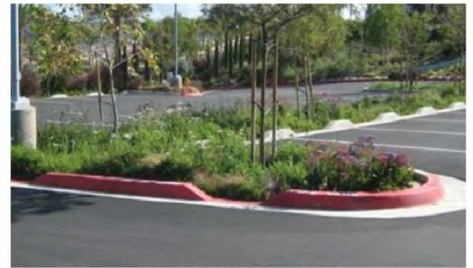
PARKING LOT BIORETENTION
