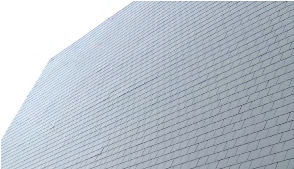
CHURCH - SLATE WALL CLADDING
