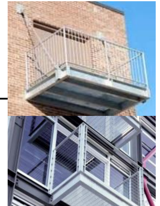
STEEL BALCONY / RAILING
