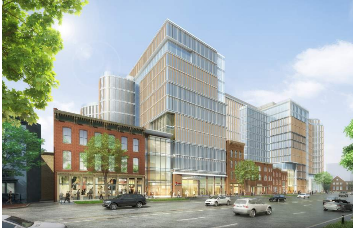
Street View along New York Avenue from Southwest
