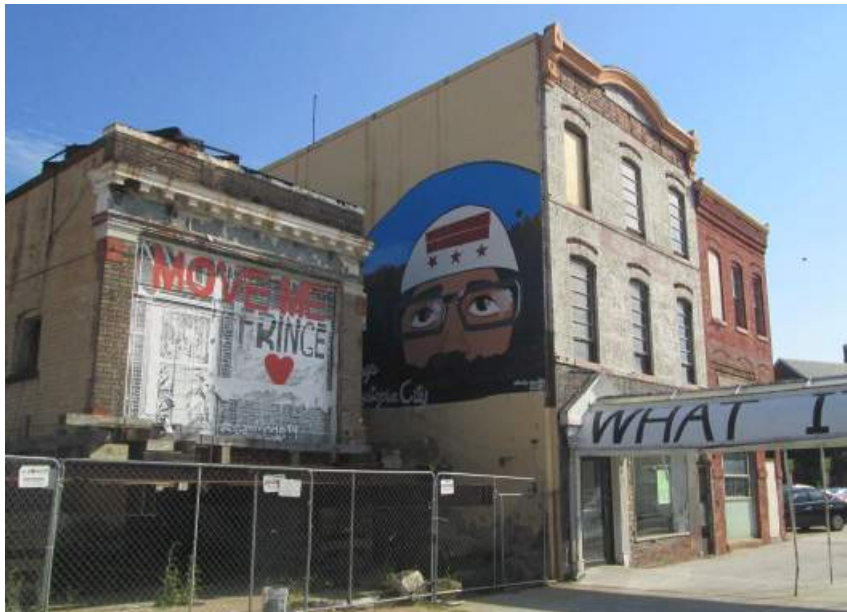
4 View from New York Avenue looking east.
