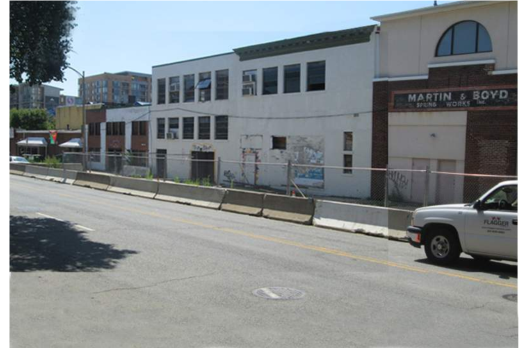
3 View from L Street looking east.
