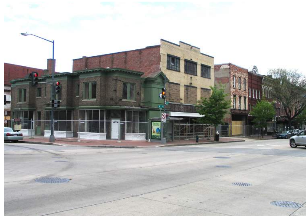
2 View from 7th and L Streets looking southeast.
