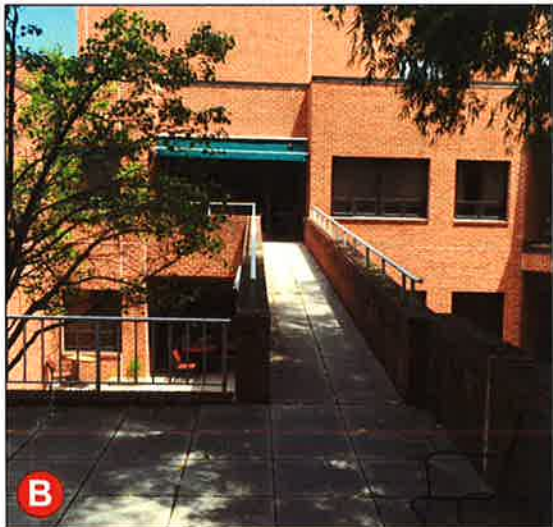
B View of Existing Bridge Looking From Tennis Courts Towards Washington Home
