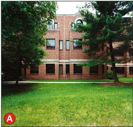
A Close Up View of Existing Facade
