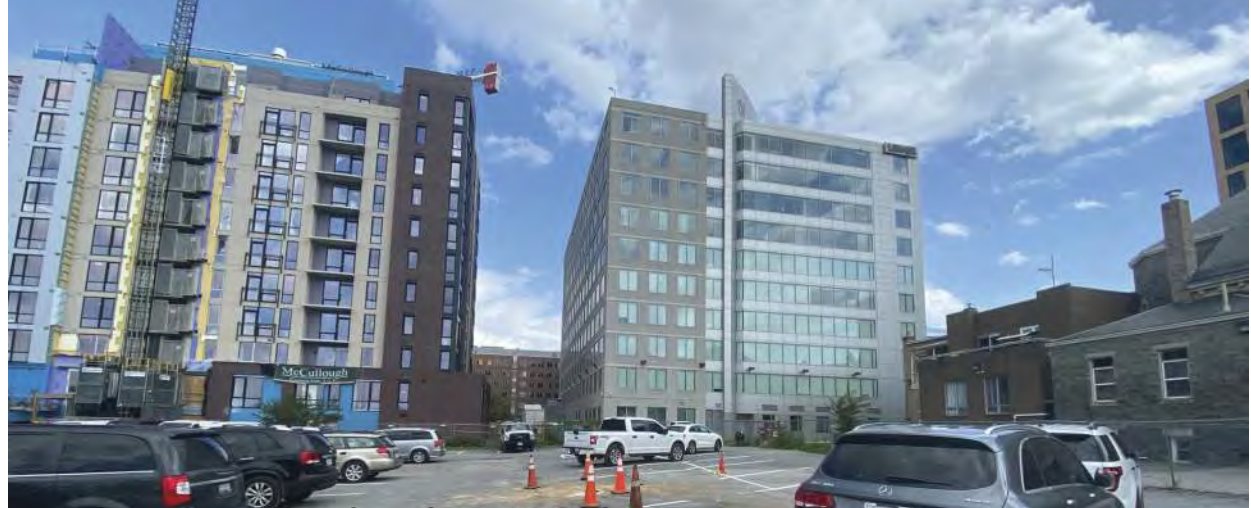
VIEW 2 - EAST NEIGHBORING BUILDINGS
