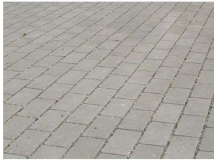
PERMEABLE PAVER TREE STRIP
