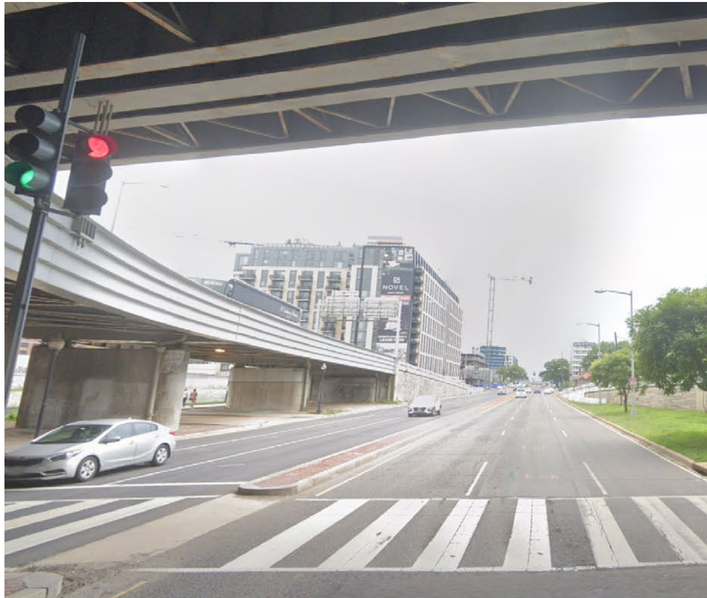
EXISTING SOUTH CAPITOL ST LOOKING SOUTH
