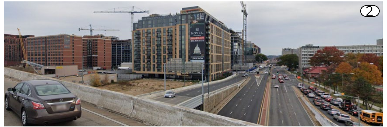
I-695 FREEWAY LOOKING SOUTH ON S. CAPITOL ST
