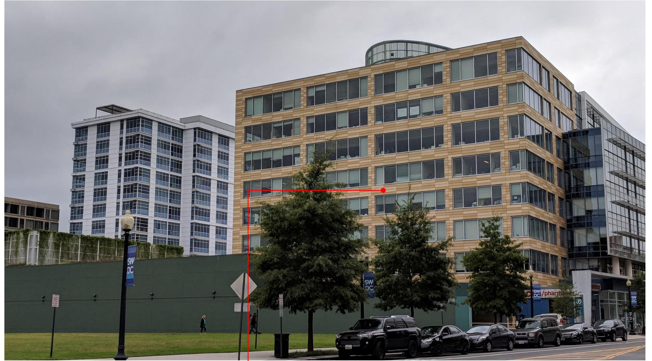
DCRA BUILDING 4TH STREET
