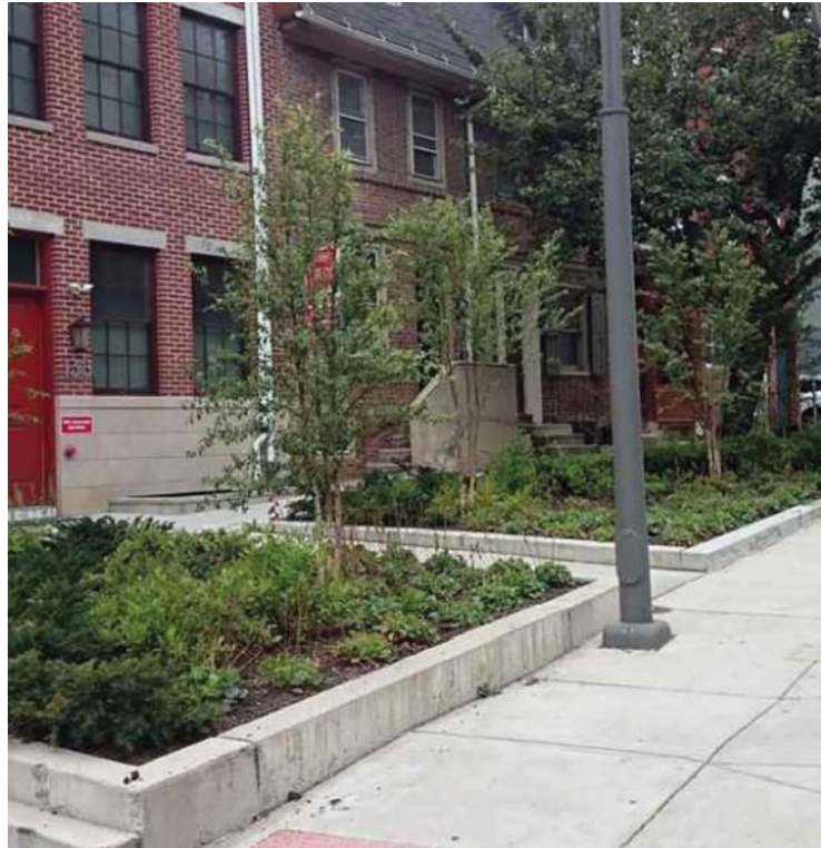
STREET PLANTINGS AND CURBED PLANTING BED
