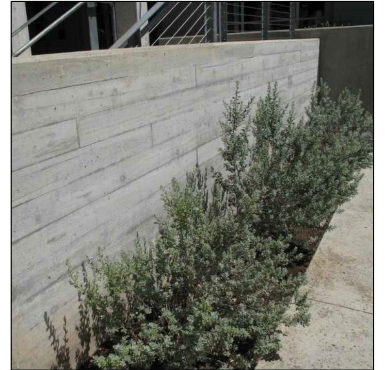
BOARD FORM CONCRETE RETAINING WALL
