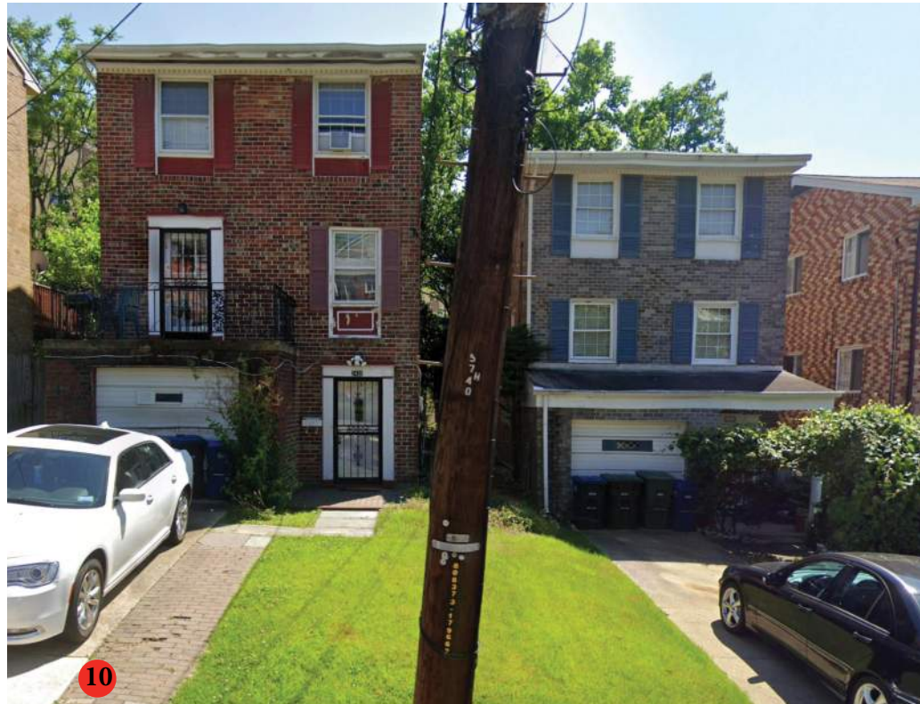
View west down Wagner St SE of Townhomes
