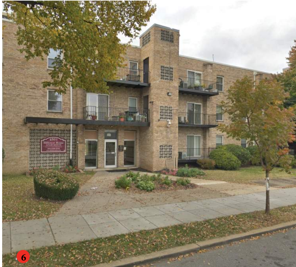
View north up 25th st SE - Hillcrest House Apartments
