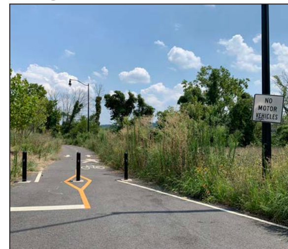
6 VIEW LOOKING NORTHEAST TOWARDS TRAIL
