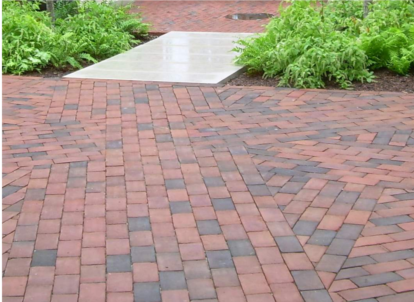
WOVEN BRICK PAVING PATTERN EPISCOPAL HIGH SCHOOL | ALEXANDRIA, VIRGINIA DESIGNED BY MICHAEL VERGASON LANDSCAPE ARCHITECTS, LTD.
