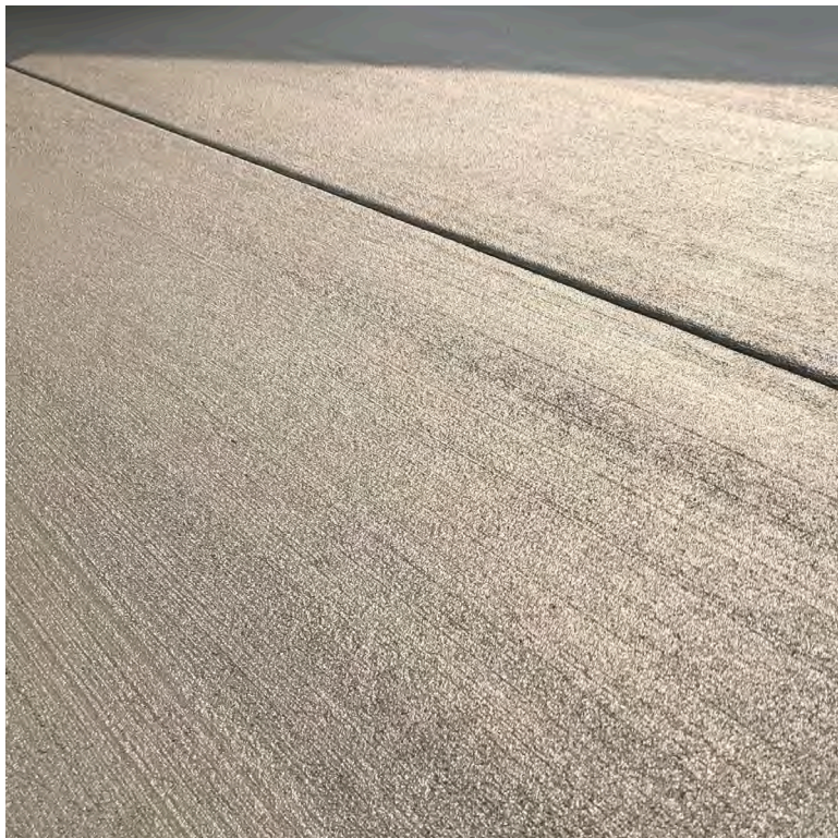
CIP CONCRETE SIDEWALK: 5' X8' Scoring, Broomed Finish
