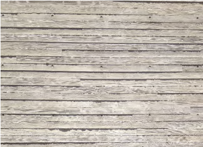
BOARD FORMED CONCRETE
