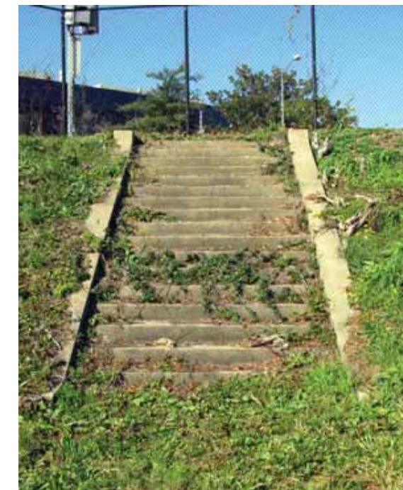
Corner stair, existing condition
