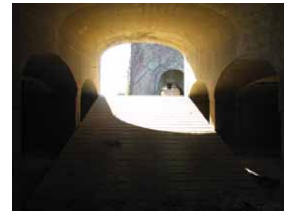
Filter bed ramp, existing condition
