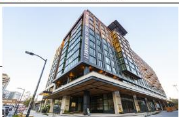
NORTH BUILDING - GABLES | EDENS
