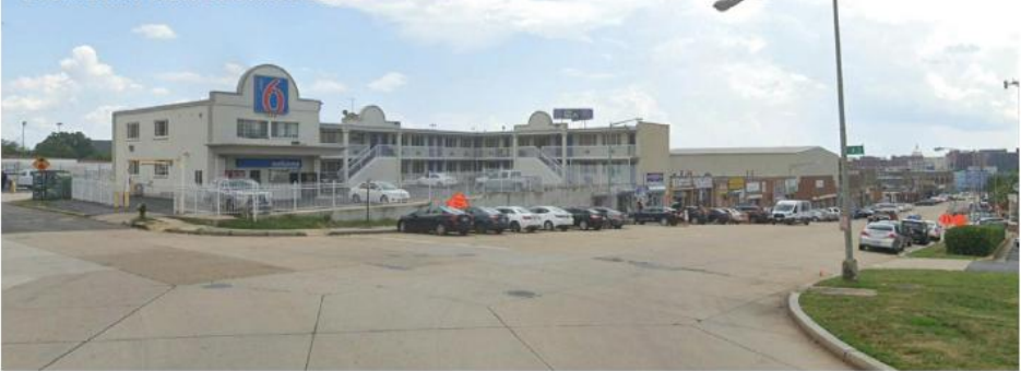
2. GATEWAY VIEW LOOKING SE
