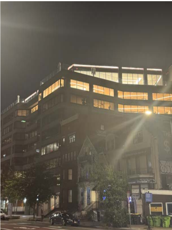
H 1919 Penn Ave Architectual Lighting
