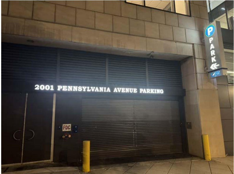
D 2001 Penn Ave Existing Parking
