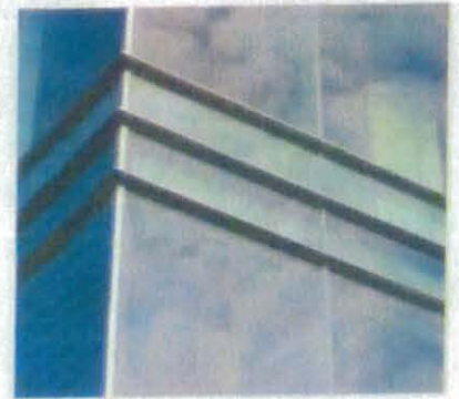
CURTAIN WALL AT PARKSIDE
