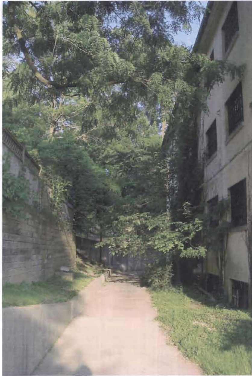
Proximity of Fraser Hall to 1630 Kalmia Road NW (Angle #1)
