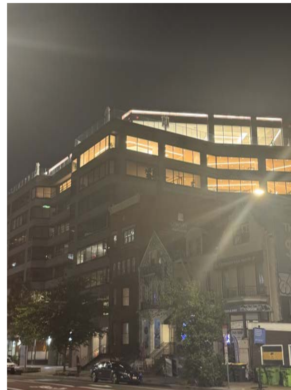
H 1919 Penn Ave Architectural Lighting
