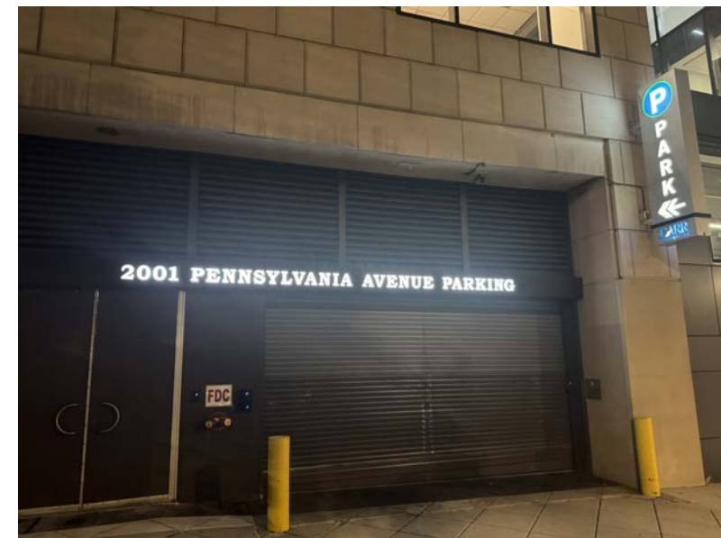
D 2001 Penn Ave Existing Parking
