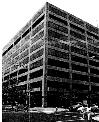
Corner of L and 21st Streets Existing
