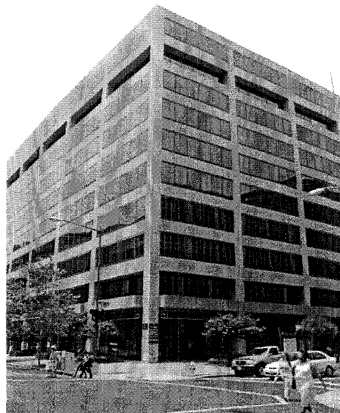
Corner of L and 21st Streets Existing
