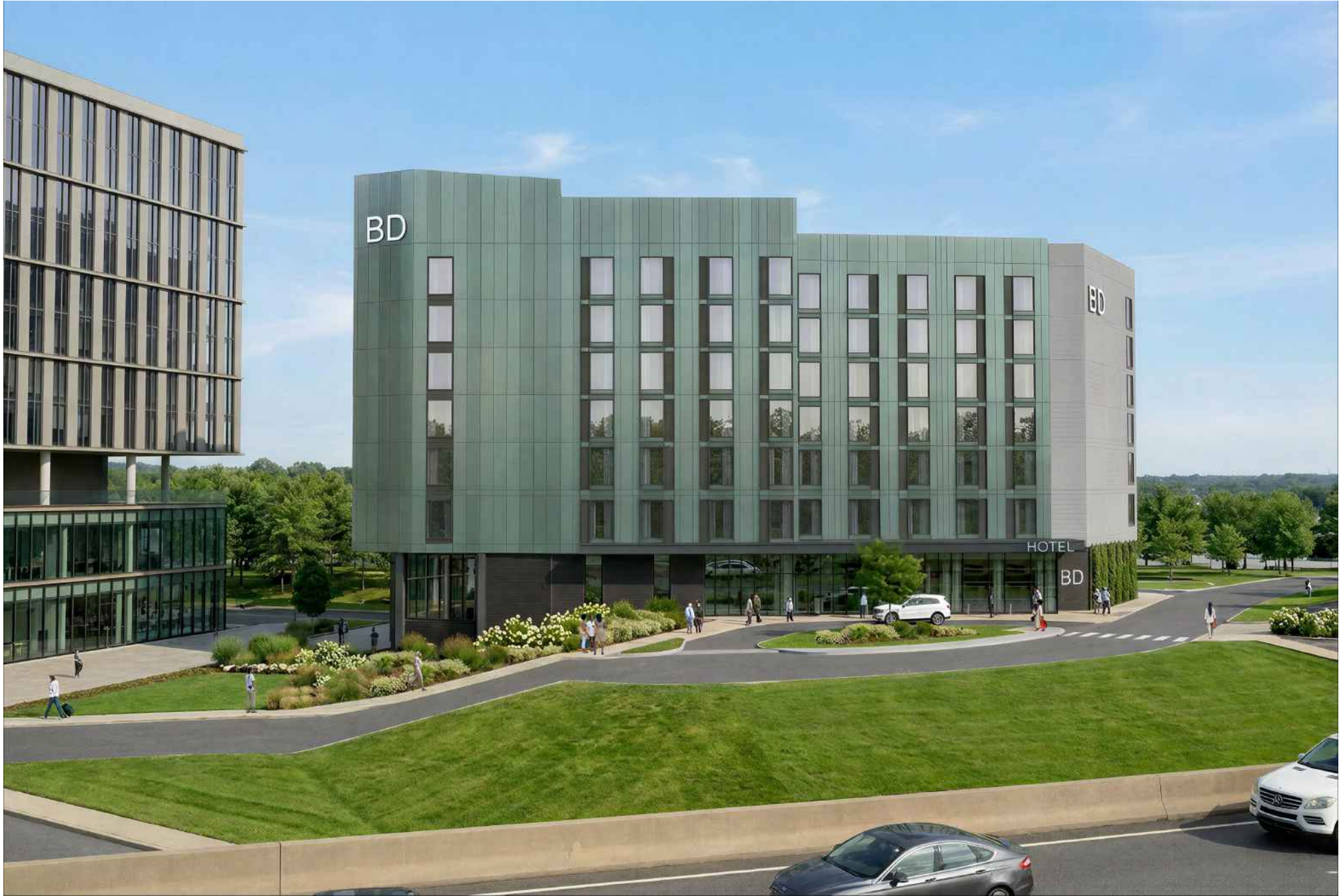
VERTICAL PANELIZATION OF GREEN FACADE PANELS
