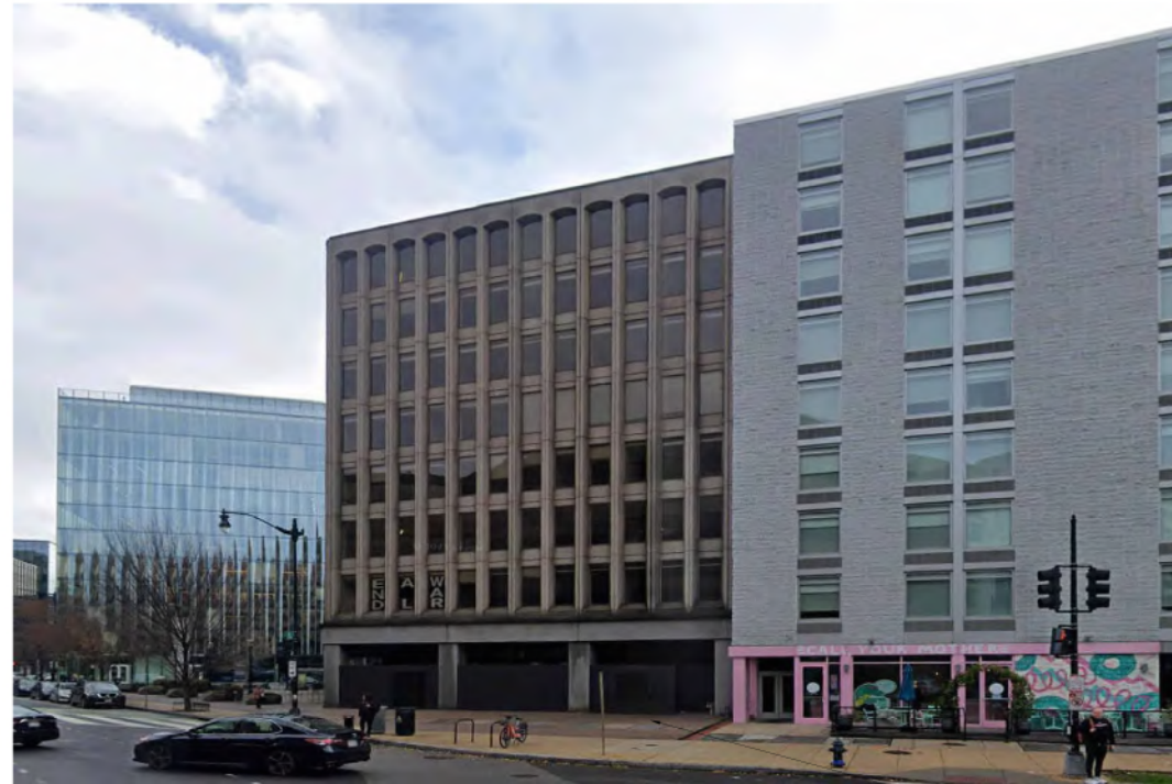
SITE PHOTO - M ST LOOKING EAST
