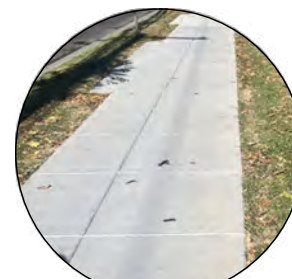
DDOT STANDARD SCORED CONCRETE SIDEWALK
