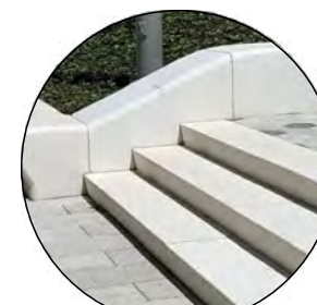
PRECAST STAIRS & TIERED SEATING
