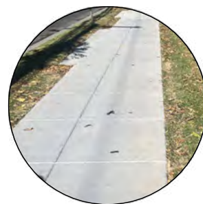
DDOT STANDARD SCORED CONCRETE SIDEWALK
