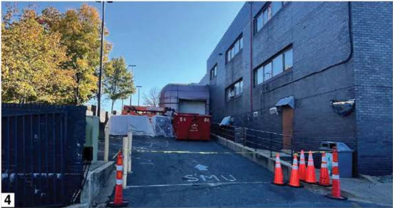
A-06 EXISTING CONDITION PHOTOS
