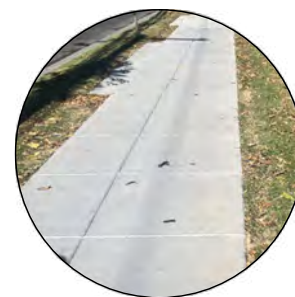
DDOT STANDARD SCORED CONCRETE SIDEWALK
