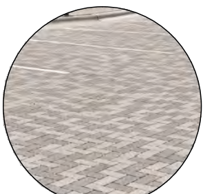
PERMEABLE VEHICULAR PAVERS
