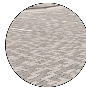
PERMEABLE VEHICULAR PAVERS
