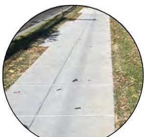
DDOT STANDARD SCORED CONCRETE SIDEWALK
