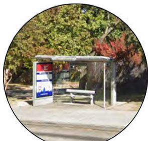
EXISTING BUS STOP SHELTER
