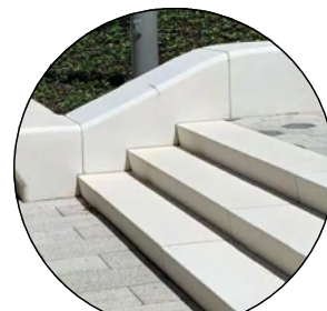
PRECAST STAIRS & TIERED SEATING
