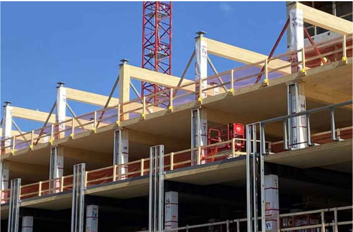
REFERENCE IMAGE: MASS TIMBER INSTALLATION
