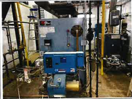
34 Boiler and steam equipment at Boiler Room 3.
