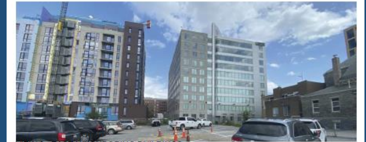
VIEW 2 - EAST NEIGHBORING BUILDINGS
