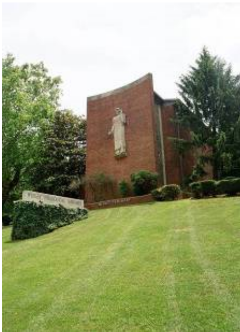
The figure of Christ on the exterior wall of the chapel facing Massachusetts Avenue was carved on site.
